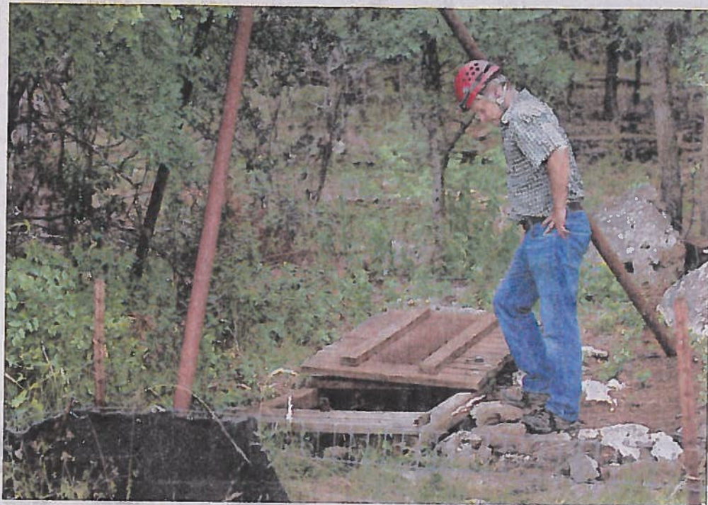
Nico Hauwert, a senior environmental scientist for Austin's Watershed Protection Department, looks at temporary wooden structures put in decades ago to help keep sediment and people out of caves in the Blowing Sink Preserve off Brodie Lane near Bowie High School. Crews will spend about two months building concrete chimneys anchored in the caves. PHOTOS BY LAURA SKELDING / AMERICAN-STATESMAN
