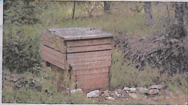
Volunteers built temporary wooden structures on sinkholes leading to the caves to keep people out, but those have since deteriorated. The structures have since plugged the entrance to some of the caves.
